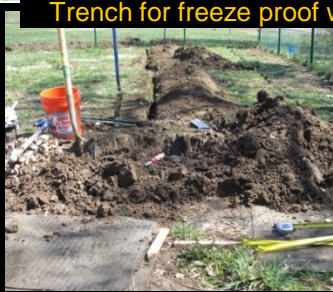
Trench for freeze proof water line
